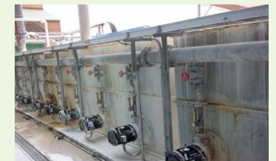
Neutralization treatment facility run by the gas emitted from the boiler
